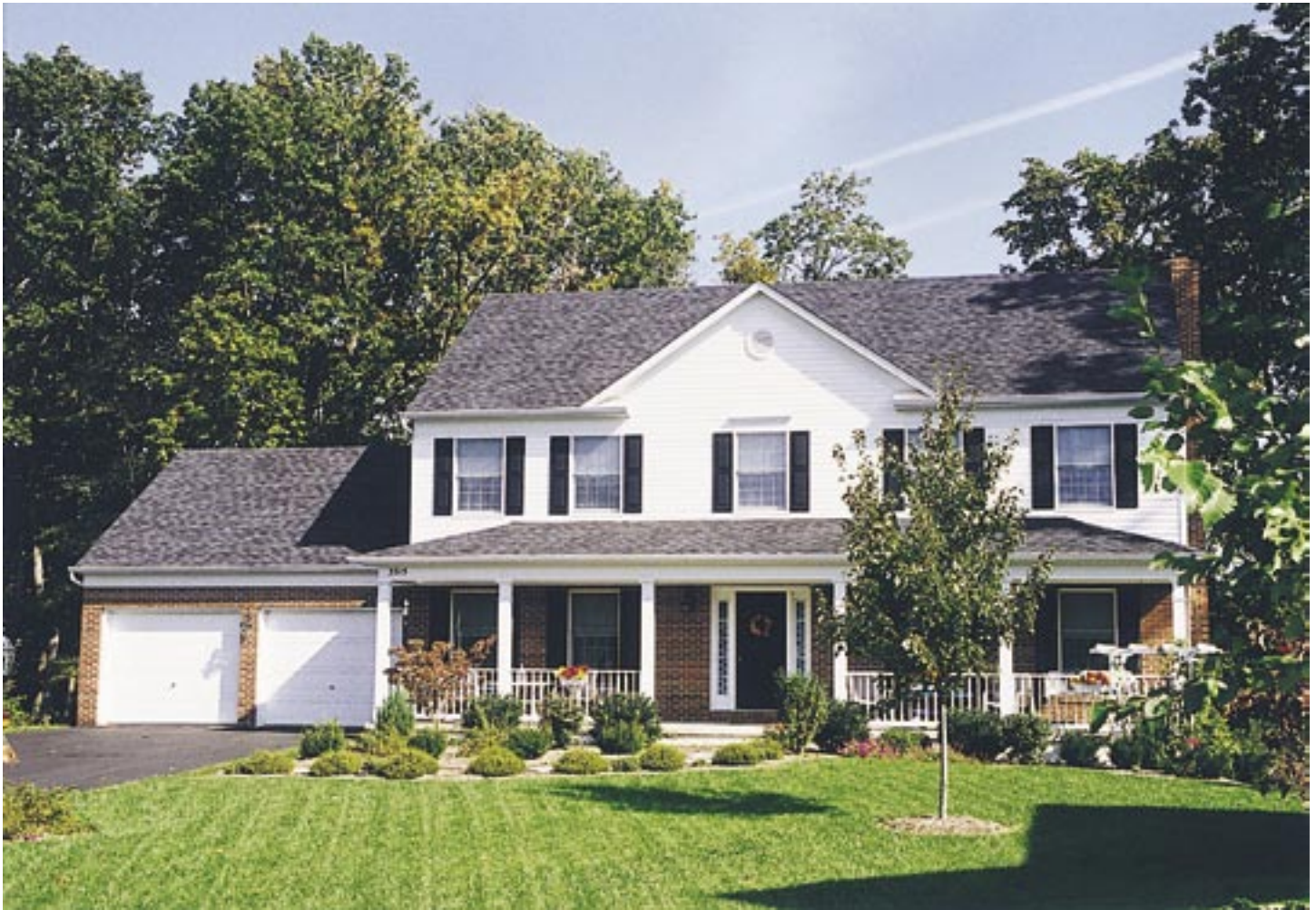
Combining convenient location with a country feel, this H.F. Payne Construction Co., Inc. home is a model of country charm. With four huge bedrooms and a well-designed lot, this home is built for today's family.
